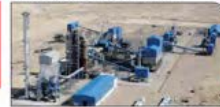
Coal based Direct Reduced Iron (DRI) / Sponge iron plant for producing high quality alternative raw material for steel making plants.
