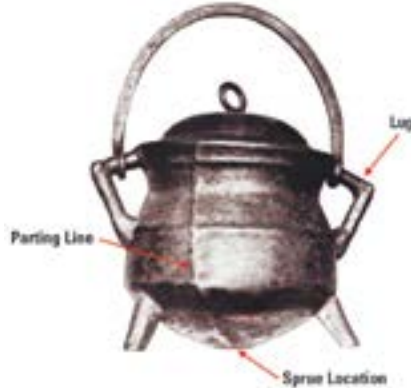
Figure 1. Photograph of the original Saugus Pot. Note prominent parting line, sprue location and handle lugs. The pot was relatively small, with a diameter of 4.5 in. and weight of about 3 lbs. with the lid. (Clyde A. Sanders and Dudley C. Gould, History Cast in Metal . Cast Metals Institute, American Foundrymen's Society, 1976, flyleaf.)
