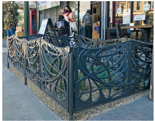
San Francisco Public Works specified this custom, cast-iron planter fence for the Upper Haight district. The intricate design captures the personality and unique aesthetic of the neighborhood, which is a blend of both French and Victorian influences combined with a counterculture vibe.
