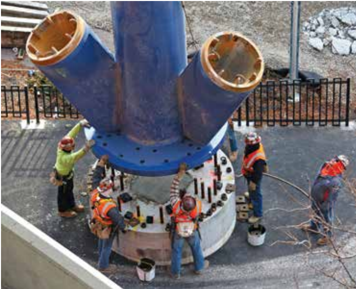
A connection is put into place outside Arthur Ashe Stadium.
