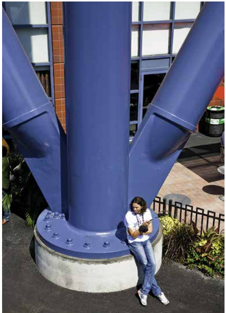
A person sits near one of the eight connections around Arthur Ashe Stadium.
