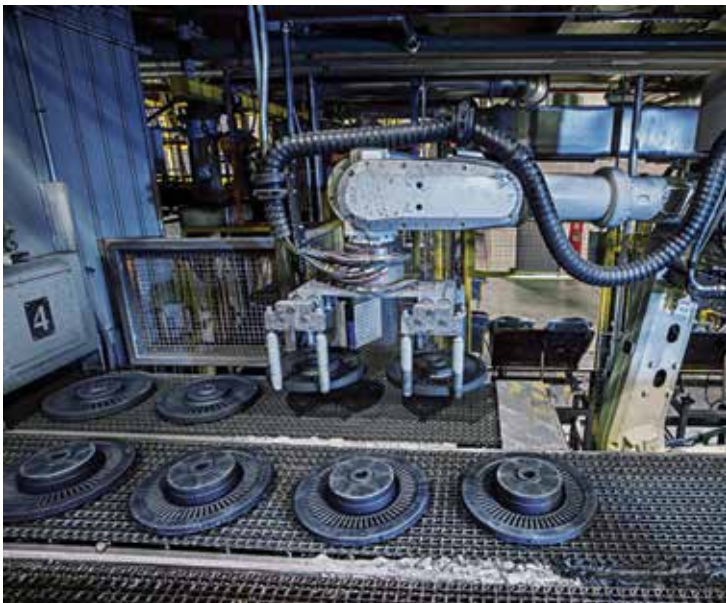
The core room at Waupaca Plant 1 underwent an extensive upgrade.
